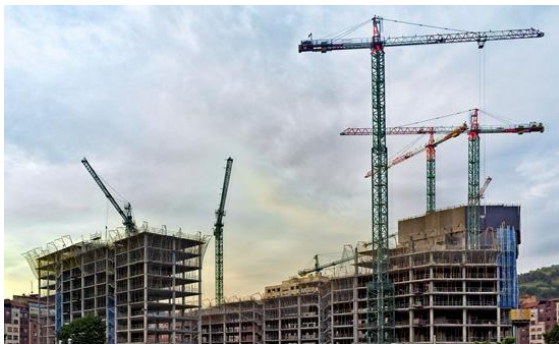
Plate 18: The Quantity Surveyor in the Construction Industry.
